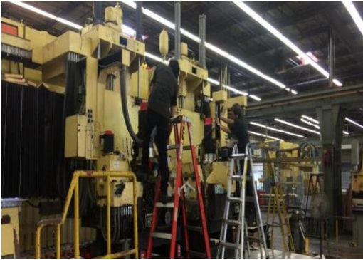
Installing new Spindle Motors to a 10 axis SNK Profiler
